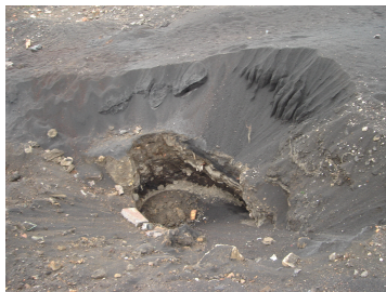
Picture 1_ remarkable depressions on the site
